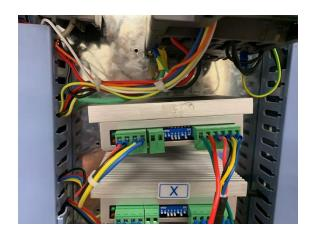
The last wiring you will need to do is to use one of your spare hole slots and feed the driver wires in and secure the connection to the outside of the cabinet as shown in the following pictures.
